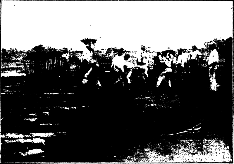
FIG. 1.—View of portion of Trinidad asphalt lake, showing digging operations. (Photo loaned by Barber Asphalt Company.)
